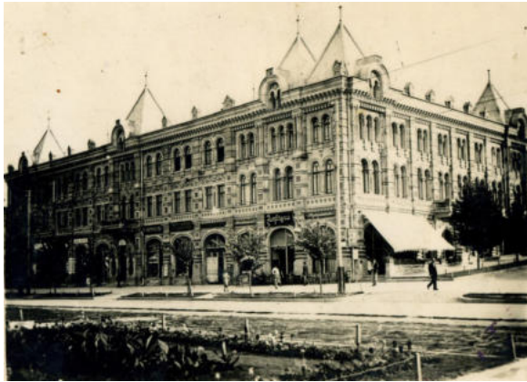
Fig. 5. Chisinau diocesan house. Architect G. Cupcea.
